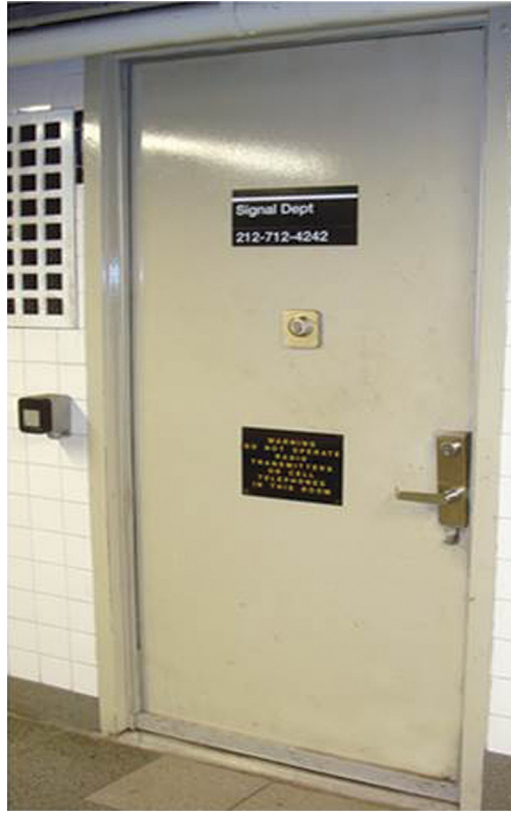
FIGURE 10.3 Linking a resistive door with electronic monitoring. This secured door to a high-voltage signal room closet is protected by two kinds of locks. The lockset is an electrically released automatic deadbolt mortise lock, released by card reader or key from the exterior and ensuring free egress at all times from the interior. A card reader is to the left. (Source: Securitech Group.)
